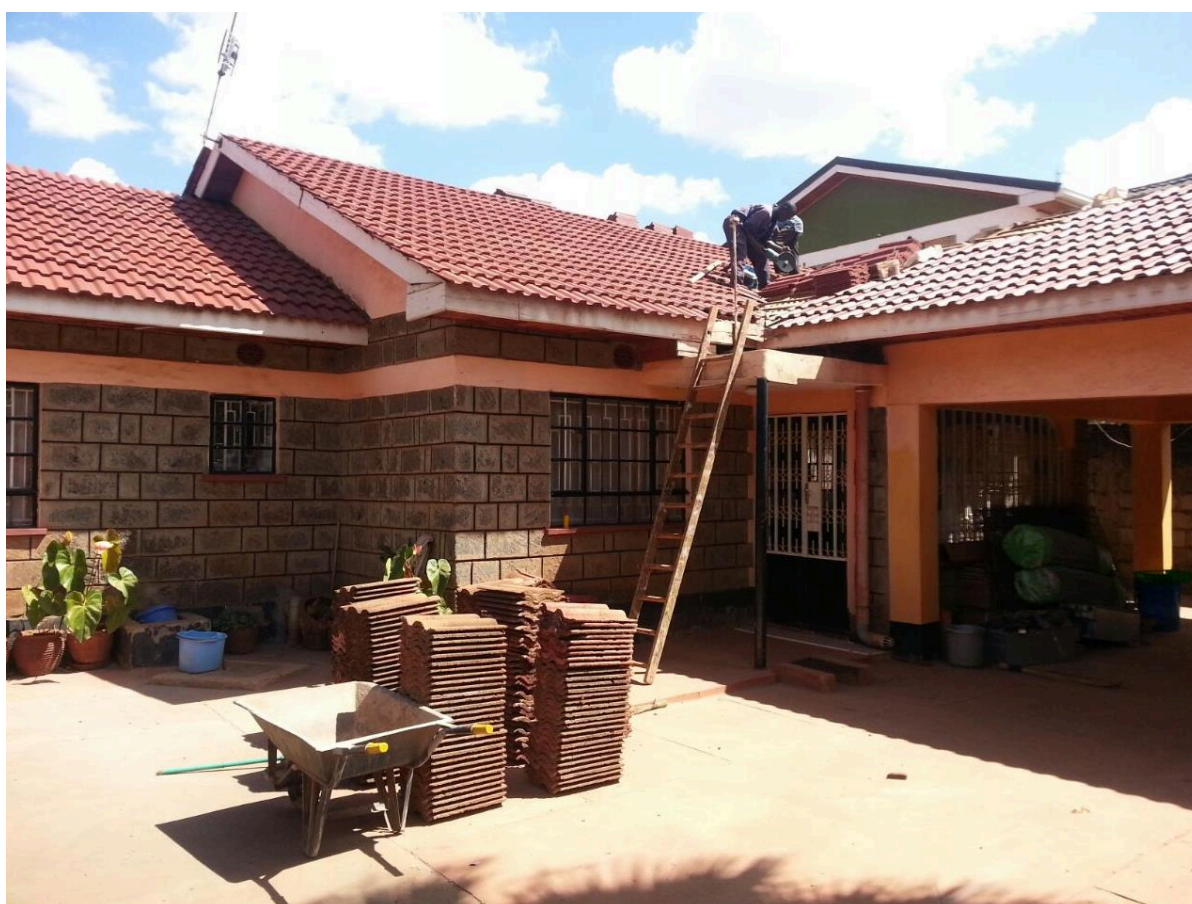
Figure 5 A roof being built with Ecoblocks and tiles.
