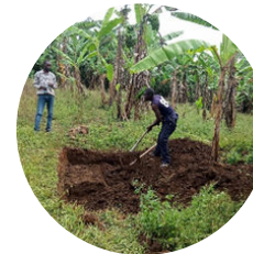
Layout and excavation
