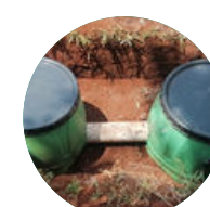
Barrel septic system
