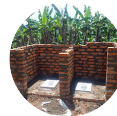
Construction of super-structure
