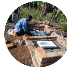
Construction of meso-structure
